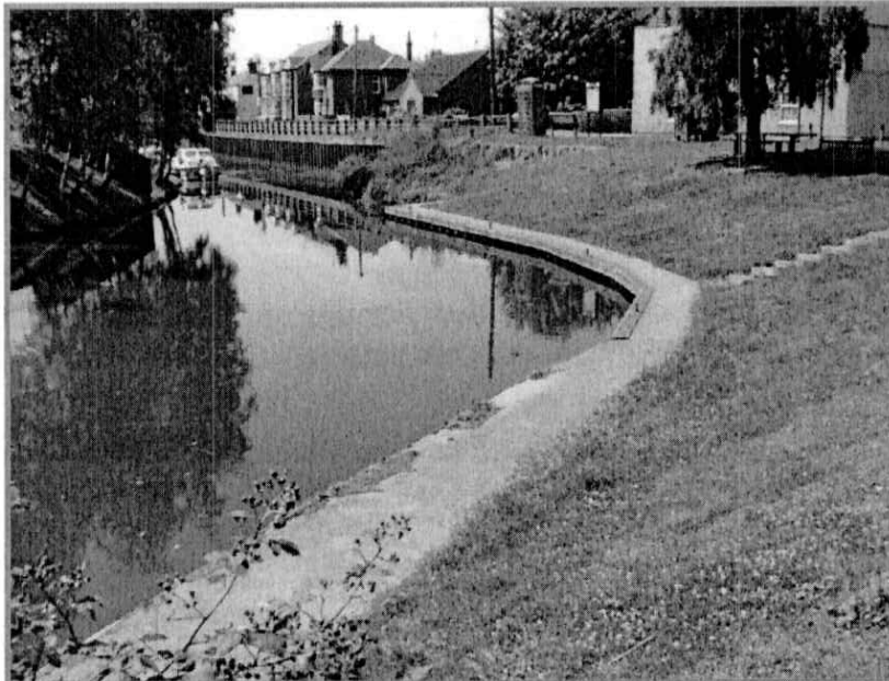
Photo 6: The boat basin, Outwell, Norfolk (application granted)
